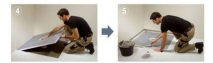
Image 1 - Measure the center of the waste area for waste cut out, cut base and then trial fitImage 2 - Apply thin-set adhesive to the floor substrate, with an 8mm notch trowel with adhesive lines running in one direction
